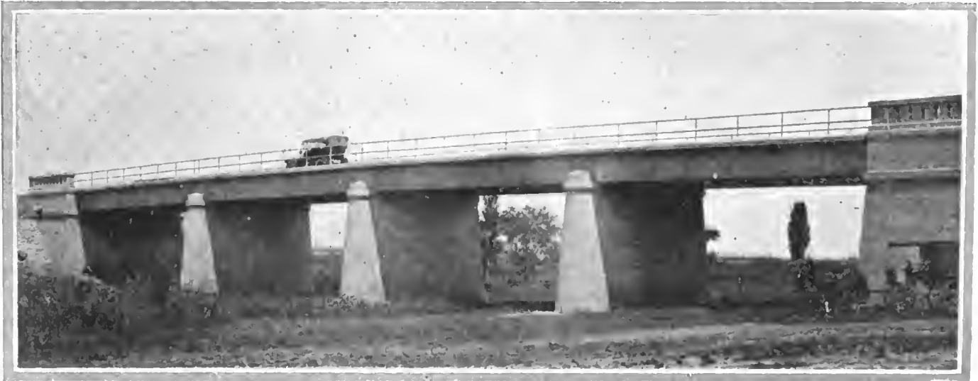
One of several examples of the high-class bridge construction being used on the new motor roads in Uruguay. This country is very ambitious in its road problems and hopes to make its roads the greatest touring fields of South America
